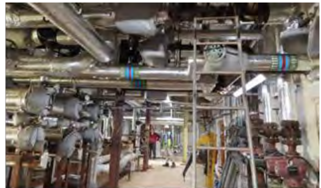
Figure 17 – Existing Plant Room
